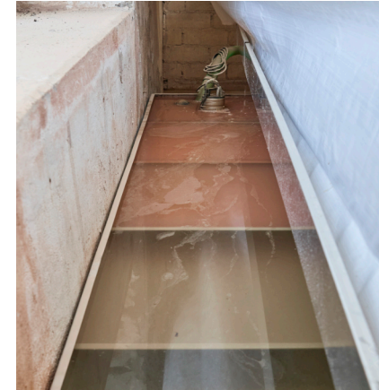
Top: Integrated water recycling system: process water is collected in settling tanks.
